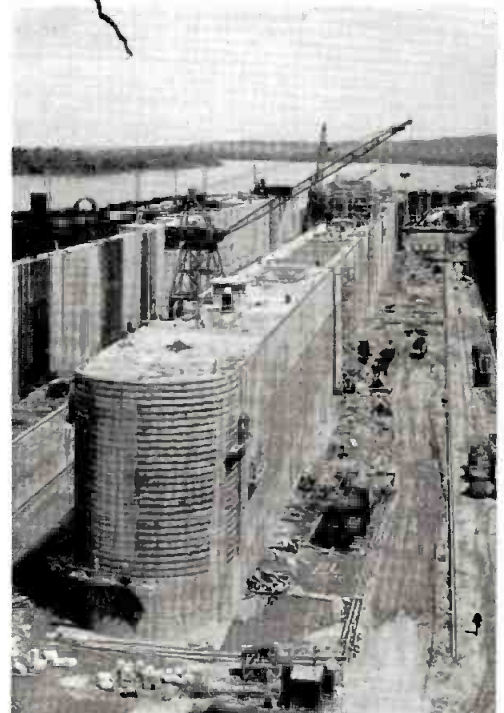
Construction view of Markland Lock and Dam — one of several under construction to handle tows longer than Queen Mary — as wide as a carrier.
